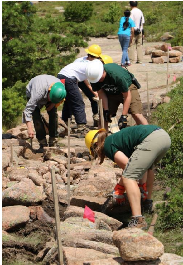
Figure 1: Setting Retaining Wall
